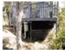
Rainwater Tanks Used to collect rainfall from all household roof areas. Stored water can then be used for toilet flushing and hot water services. Design issues include sizing tanks for reliable supply and incorporating tanks into urban design.
