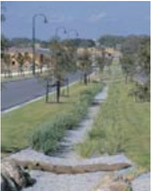
Bioretention System for Valley Connector. Typical width of 3 to 4 m with roads on either side having a single crossfall towards the bioretention system. The example pictured incorporates use of a gravel filter medium. A fully vegetated surface with filtration through sandy loam is recommended unless pre-treatment for coarse and medium sediments can be ensured through the use of grass buffers.
