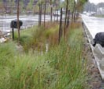
Similar to Valley Connector bioretention type 2, but used where grades are flat and catchment areas are smaller (where flow capacity and conveyance are less of a design issue). Runoff is detained in a manner approaching treatment within a 'raingarden'; with dense vegetation and a disconnected flow path.
